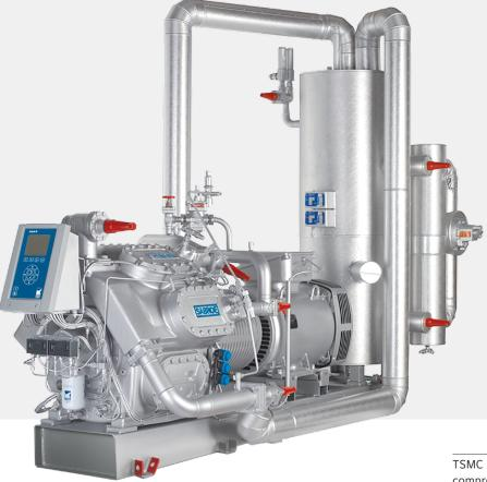
TSMC 108 two-stage reciprocating compresor unit shown with closed flash inter-stage cooling system and UniSAB systems controller
